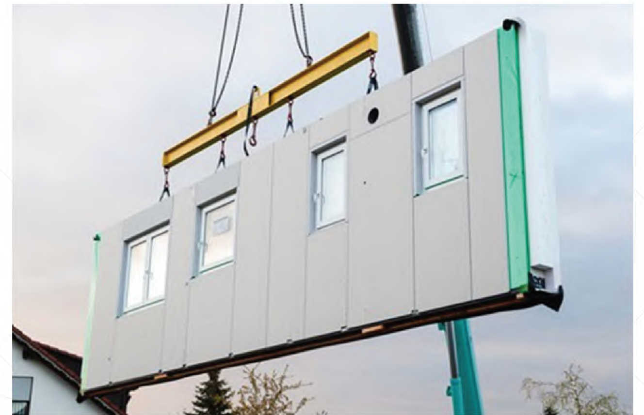
Figure 2.16. Example of Panellised
