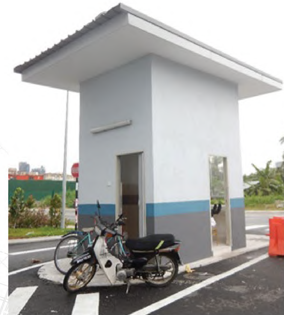
Figure 1.8. A security post located at the entrance of a residential premise
