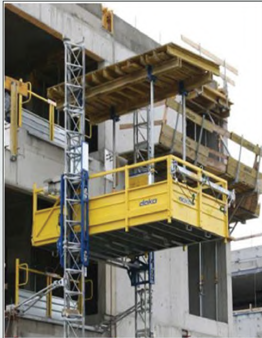
Figure 2.9. DOKA Lifting System to lift a table formwork (Kang, 2013)
